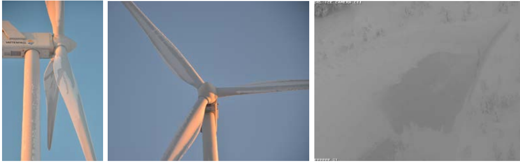
Figure 18: Ice creation on wind turbines in Stor-Rotliden, February 2019.
